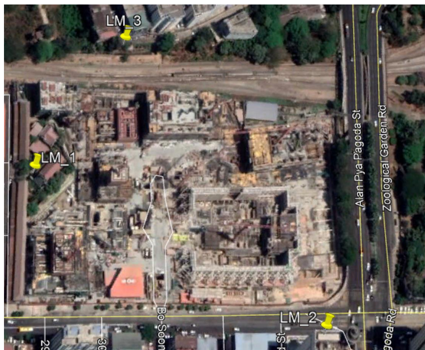
Figure 4-1 Air monitoring point around YCP
